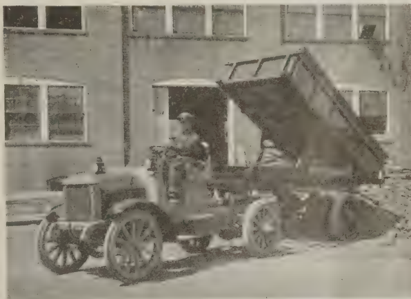
A LIGHT-DUTY TRACTOR WITH HAND-OPERATING SEMI-TRAILER.
